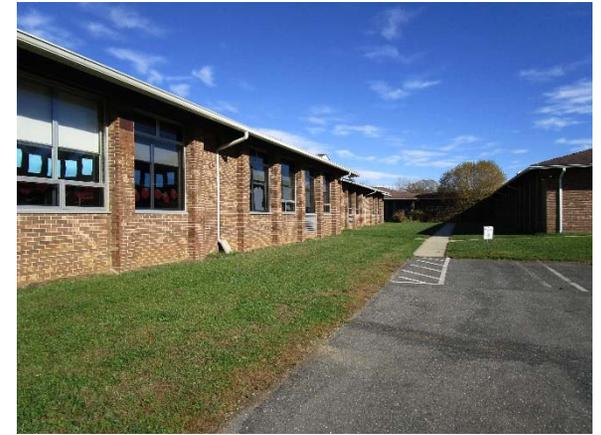
Installing rain gardens adjacent to the building and by the parking lot can capture, treat, and infiltrate roof runoff. A rain garden near the parking lot can help remediate some of the erosion occurring and capture runoff from the parking lot. A preliminary soil assessment suggests that the soils have suitable drainage characteristics for green infrastructure.
