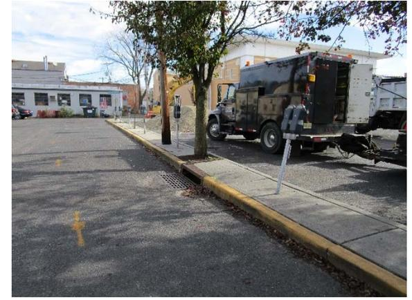
Parking spots along the street can be replaced with porous asphalt to capture and infiltrate stormwater. A preliminary soil assessment suggests that more soil testing would be required before determining the soil's suitability for green infrastructure.
