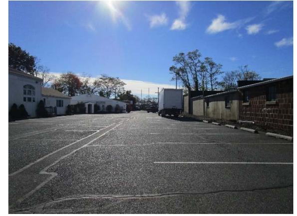
Parking spots can be replaced with porous asphalt to capture and infiltrate stormwater from the parking lot and rooftop by directing downspouts into it. A preliminary soil assessment suggests that the soils have suitable drainage characteristics for green infrastructure.
