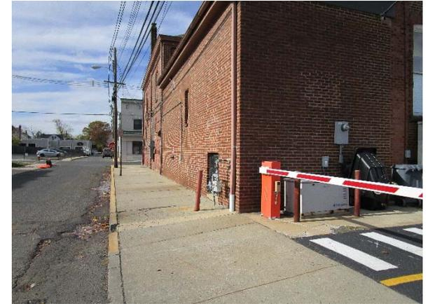
Installing a rain garden adjacent to the building can capture, treat, and infiltrate roof runoff. A stormwater planter can be constructed to the south of the building by directing the downspout that is already routed under the sidewalk into the planter. A preliminary soil assessment suggests that more soil testing would be required before determining the soil's suitability for green infrastructure.
