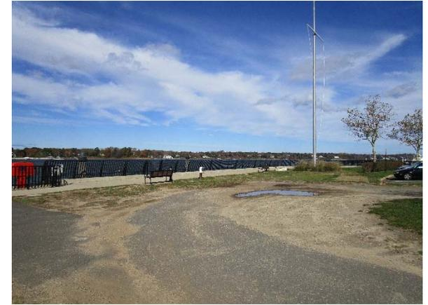
Parking spots to the north end can be replaced with porous asphalt to capture and infiltrate stormwater. Installing rain gardens in the eroded areas around the park can capture, treat, and infiltrate runoff from the parking lot and walkways. A preliminary soil assessment suggests that the soils have suitable drainage characteristics for green infrastructure.
